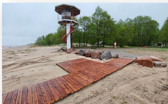
Figure 27. Wooden boardwalk installed during the project on Kabli Beach
